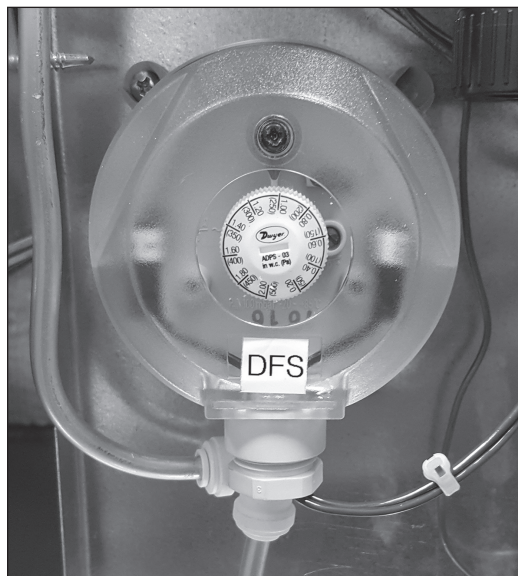
Figure 26.3 - Dirty Filter Pressure Switch
