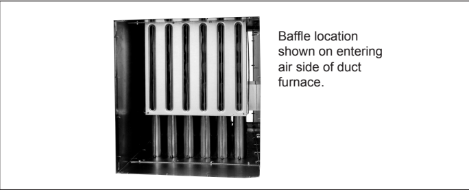
Figure 4.1 - Air Distribution Baffle Location
