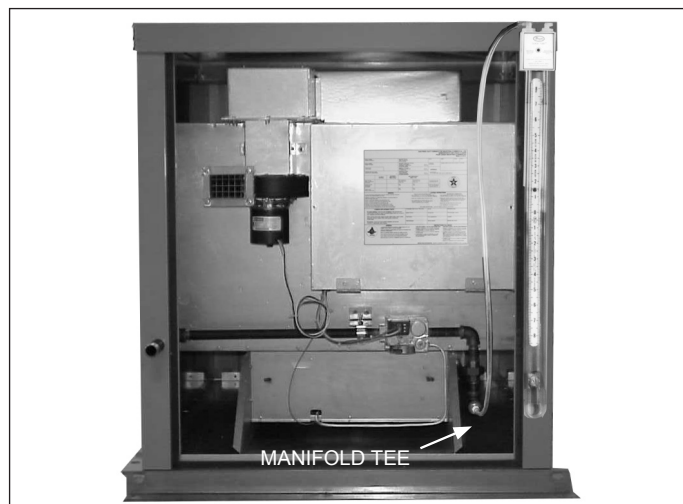
Figure 15.2 - Maxitrol Modulating Valve Adjustments
